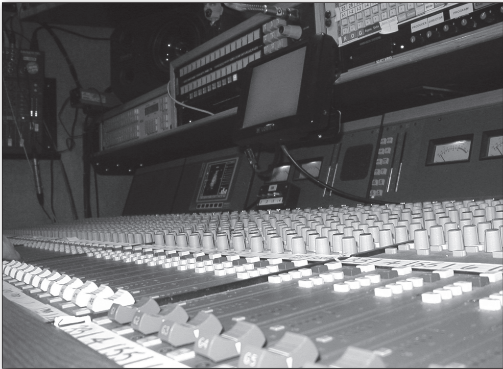
Figure 1.2 The mixing console is the control center for all audio signals.
